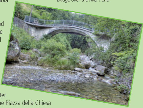
Bridge over the river Perlo
